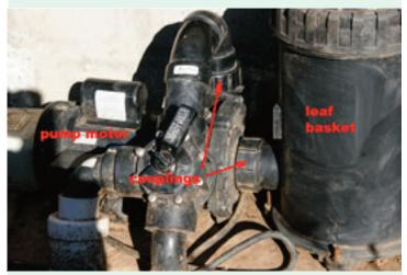
My tool of choice for this task is a strap wrench. They're readily available, will fit nearly any size fitting, are inexpensive, and won't damage what you're trying to turn. Don't forget to set the inlet and outlet valves to "off" and unplug the pump before you begin.
