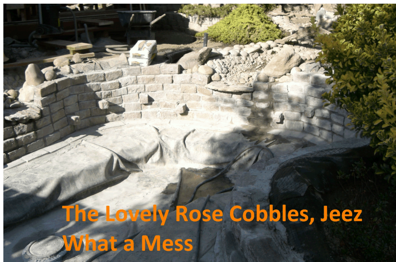
Cobble Wall In Place
