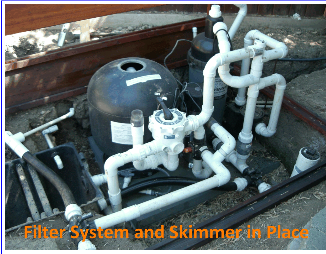
Vaunted Bead Filter and Turbo Vortex
