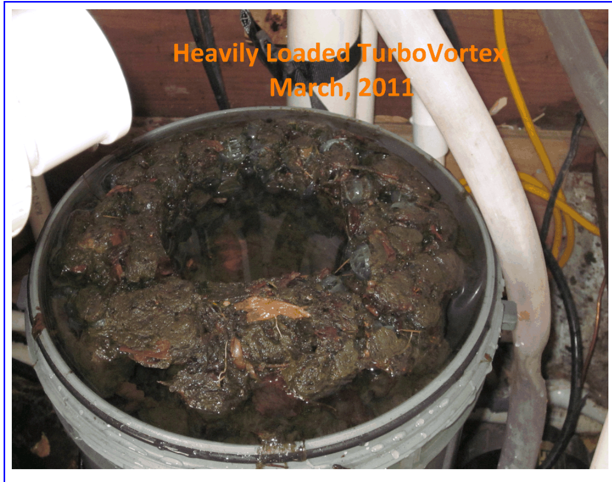
A Plugged Up Turbo Vortex
